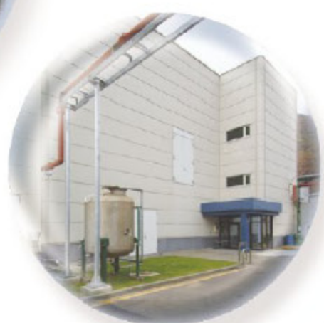
Capsulation facility (Ueda Plant)
